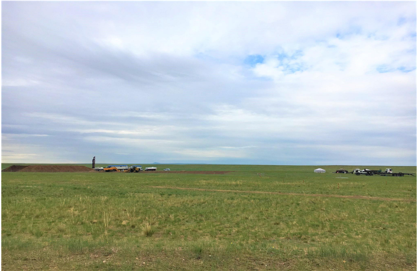
Red Deer 1 site under construction. Water supply well drilling
